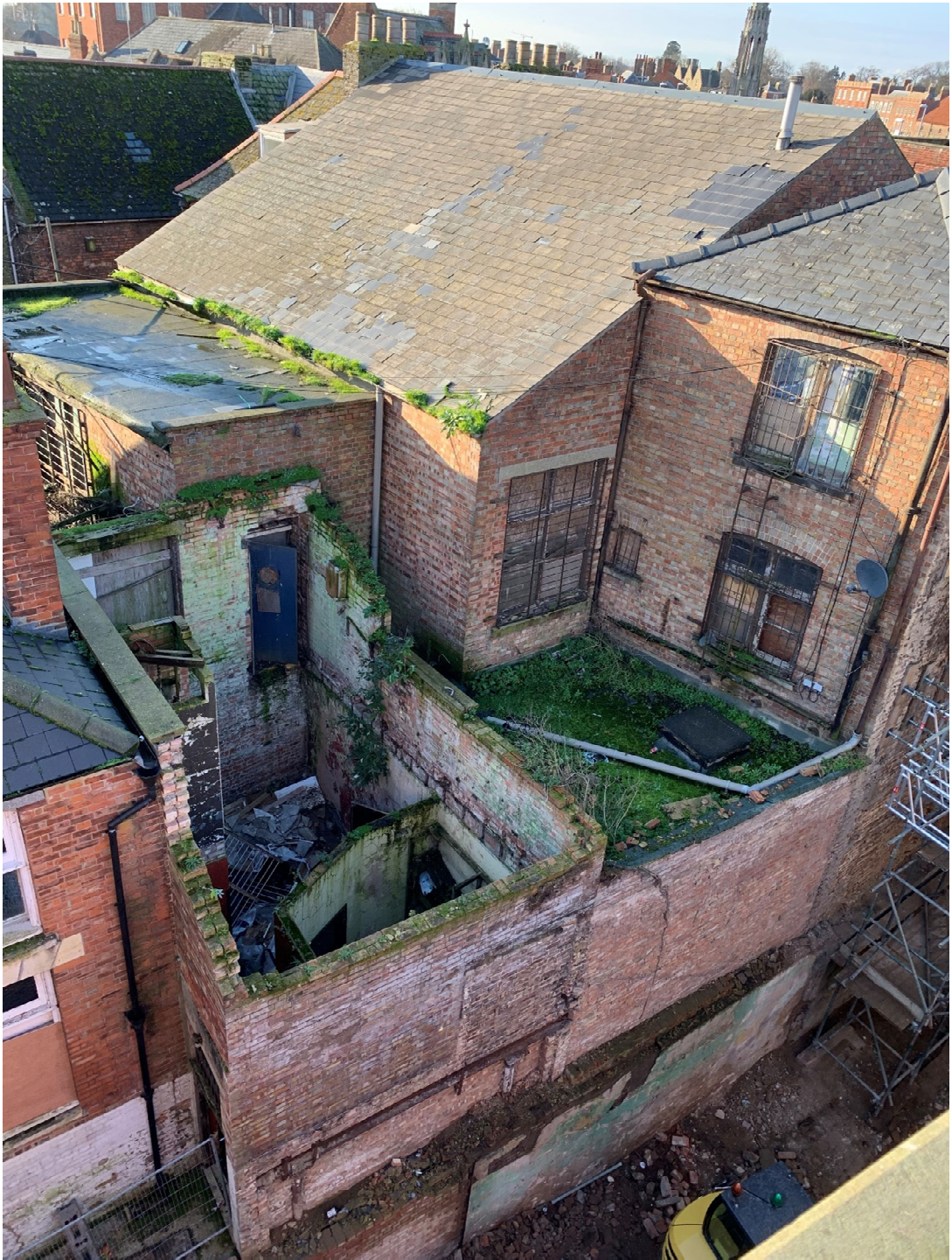
Rear of 13-17 High St as viewed from No 10 – November 2020
