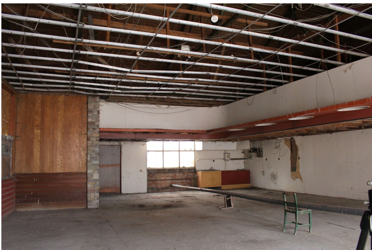
13-17 High Street 1 st floor interior – 2018
