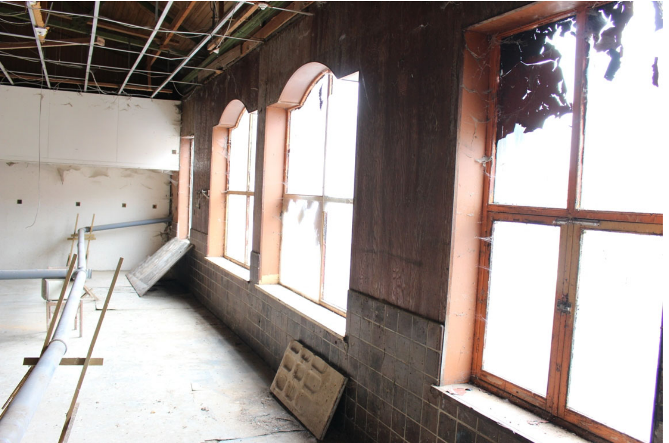
13-17 High Street 1 st floor interior – 2018
